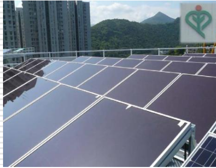
Thin-film silicon solar cell unit 硅薄膜太阳能电池组件 (Architectural Services Department 建筑署)
